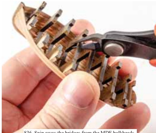
836. Snip away the bridges from the MDF bulkheads.
