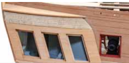
478. Glue the 3mm parts together while temporarily sitting them underneath the quarter galleries. When set, sand to profile as shown and fit to the hull. The 1mm parts need to be carefully shaped so they just overhang the roof, and the outer edge rounded off. Glue to the model.
